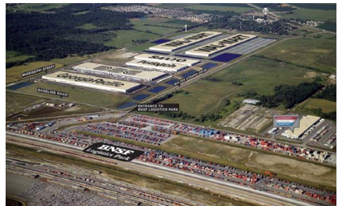
Logistics Park Chicago, also known as CenterPoint Intermodal Center, is a major ILC in the far Southwest suburbs of Chicago.
