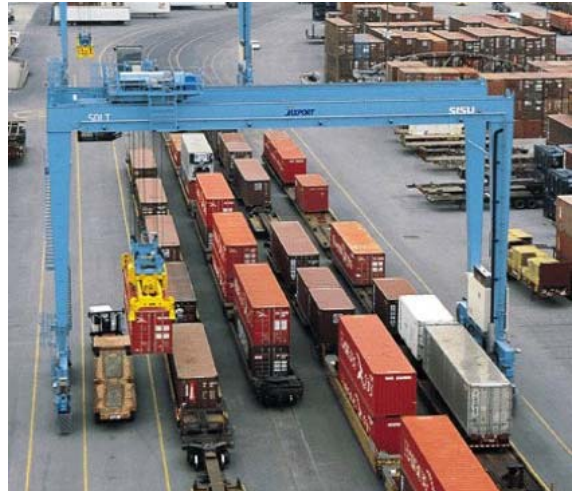
This image illustrates how shipping containers are moved from trucks to train cars at an intermodal facility, also known as a “ramp.”
