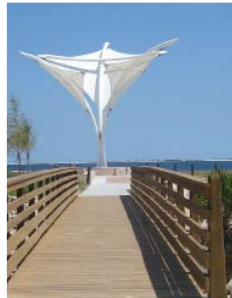
The spires and fabric wings of this structure (top, during construction; above, completed) were designed by ValleyCrest Design Group/SiteWorks Studio to emulate flight and the flying spirit of the U.S. Navy. Serving as a focal point in the west plaza of the Pensacola Naval Air Station, the sculptural feature was engineered and installed by Fabric Architecture of England.
