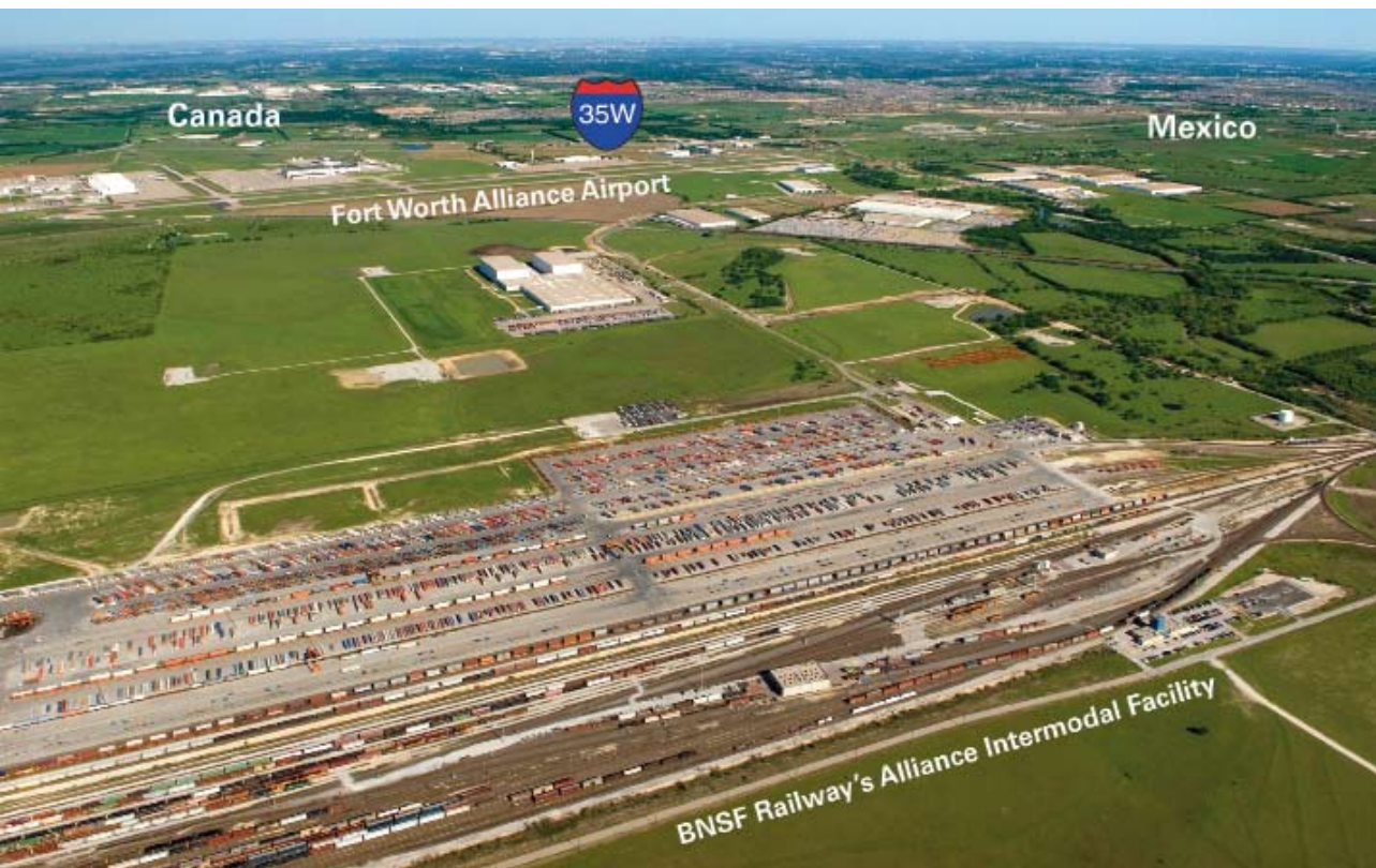
The AllianceTexas logistics hub, which features a Burlington Northern Santa Fe intermodal facility, is conveniently located near both Fort Worth Alliance Airport and Interstate 35.
