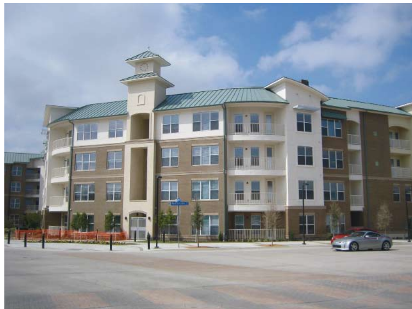
The Venue, a 279-unit apartment complex under construction, is part of a transit-oriented development taking shape near the Galatyn Park Station in Dallas.
