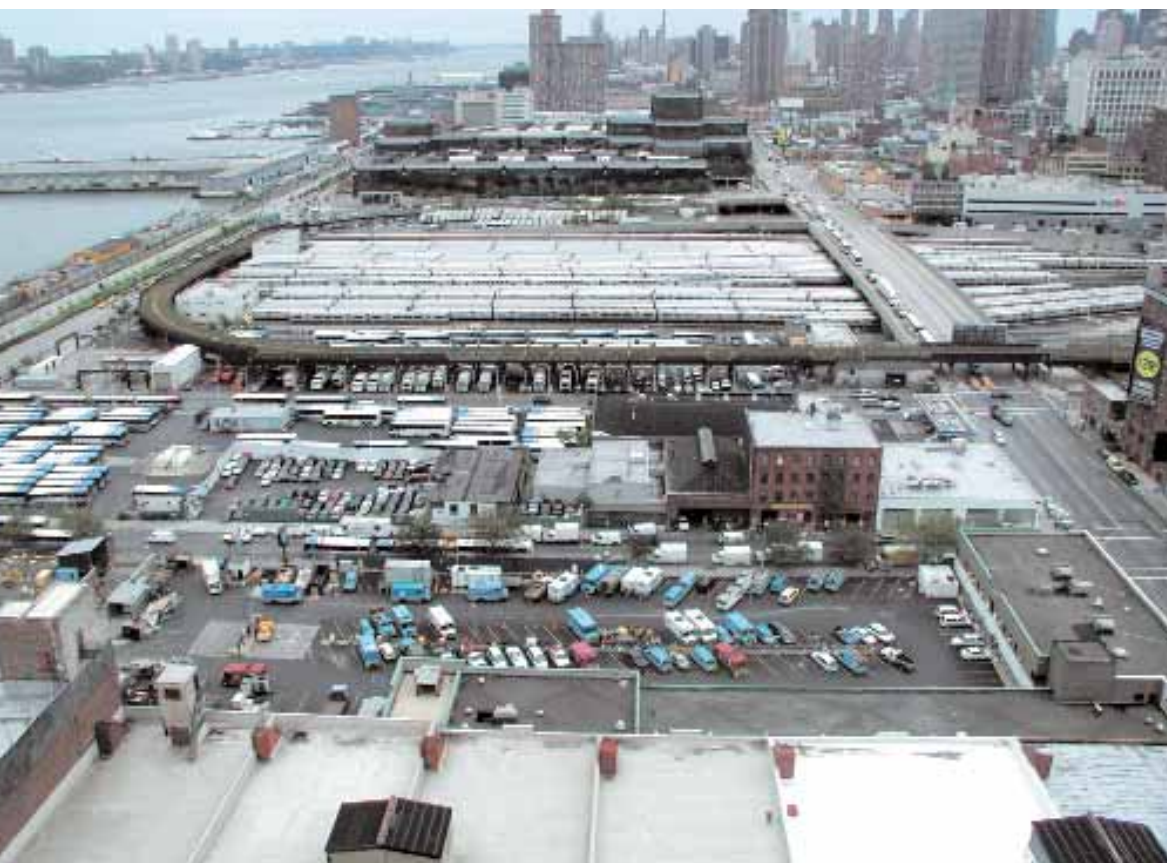
The proposed New York Sports and Convention Center stadium will rise above the existing Long Island Rail Road storage yard. The rail yard is currently below grade and would be decked over to construct the stadium, as well as 5 million square feet of development and six acres of open space, while maintaining its current use below.
